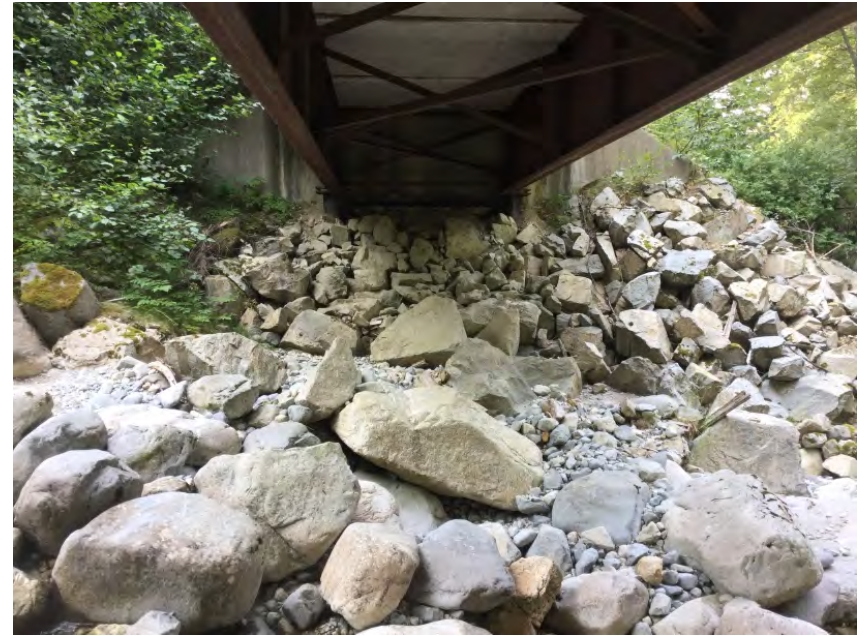
Left Bank Abutment when facing downstream
