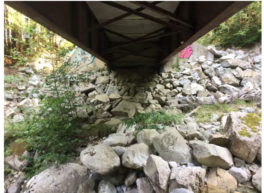
Right Bank Abutment when facing downstream
